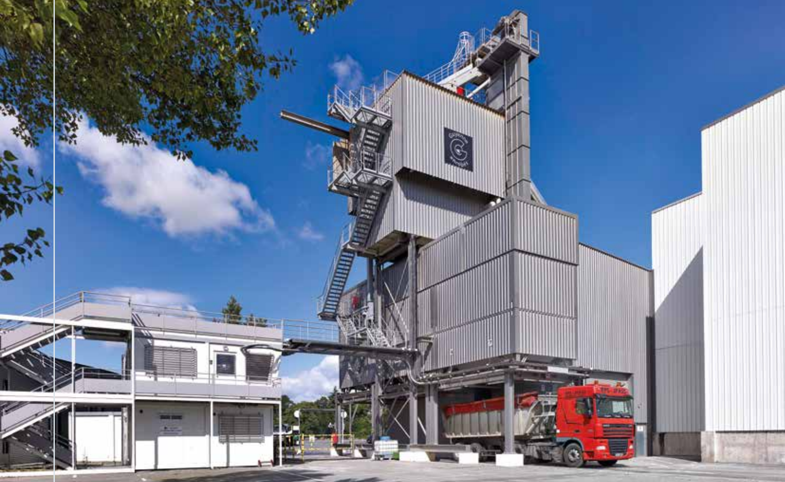
Photo above: The Universal produces approx. 30000 t low temperature asphalt per year – that is about \frac{1}{3} of its annual production. Photo under: The Universal is the classic among asphalt mixing plants in Europe – a versatile plant with high capacity. High additions of recycling are also possible via the parallel drum.
