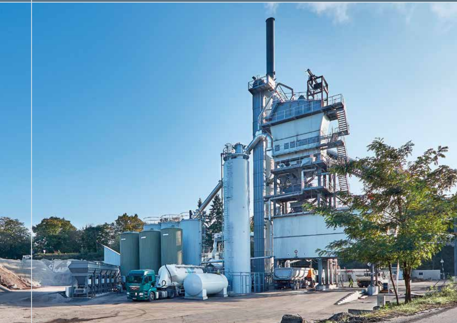
Photo above: The Universal produces approx. 30000 t low temperature asphalt per year – that is about \frac{1}{3} of its annual production. Photo under: The Universal is the classic among asphalt mixing plants in Europe – a versatile plant with high capacity. High additions of recycling are also possible via the parallel drum.
