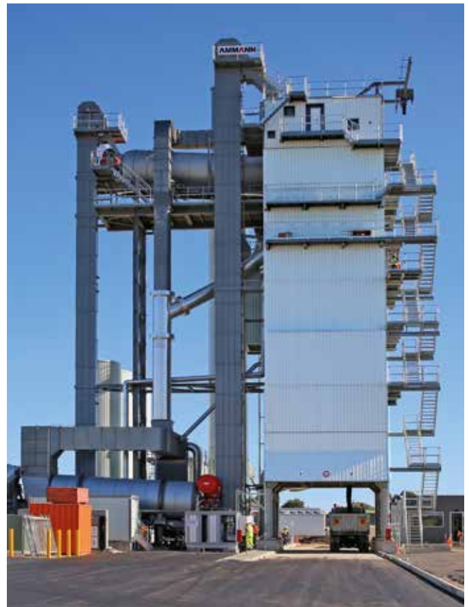
The Universal HRT with clad tower and equipped with a parallel drum for the recycling addition up to 60%.
