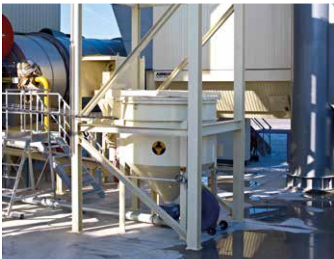
Addition of additives (granulate).
