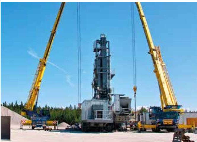
A considerable advantage of assembly on site: The elevators (filler and hot elevator) and the bitumen pump are preassembled together with the chassis and form a solid unit all together.
