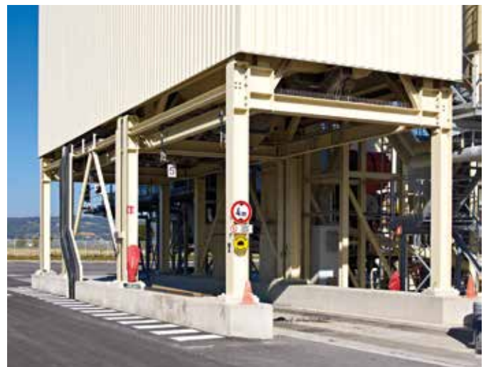
Single-track hot mix storage silo in throughput direction.
