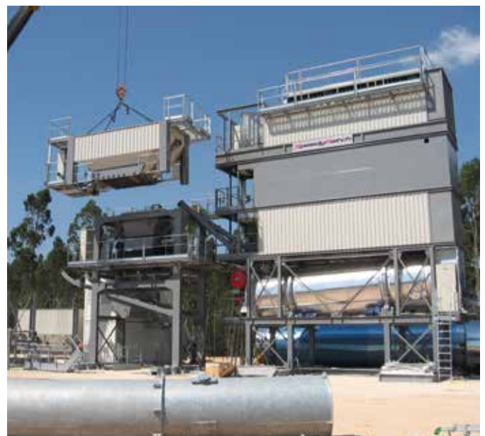
A firm compacted base is sufficient for erecting a SpeedyBatch.
