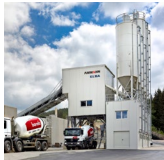
Concrete mixing plants
